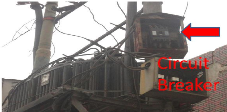
Figure 07. PMTs with circuit breaker. SOURCE: visit to HESCO
