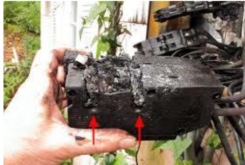
Figure 02. Burnt circuit breaker
